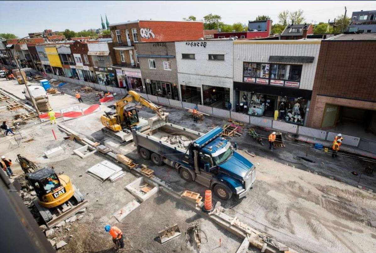
**EXCAVATION**: REMPLACEMENT AVEC TRANCHÉE OUVERTE
